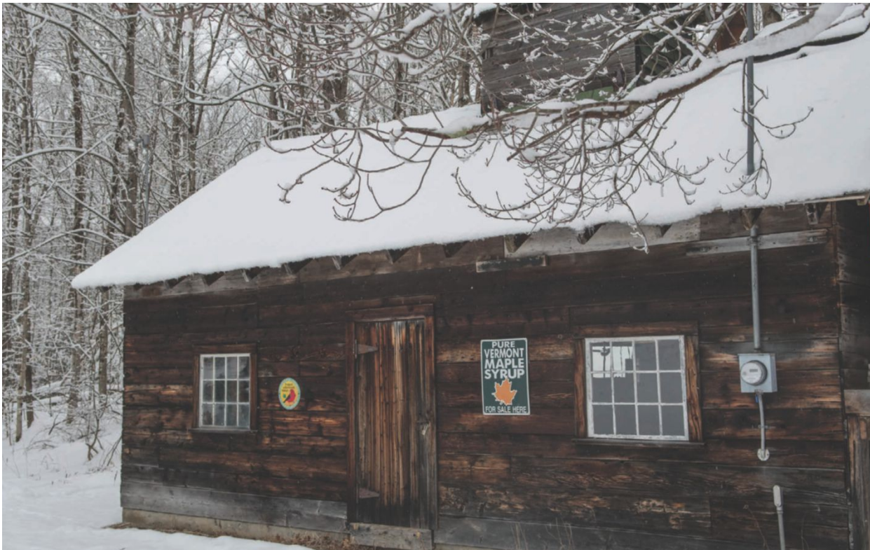
THE GREEN MOUNTAIN AUDUBON CENTER IN HUNTINGTON, VT.
